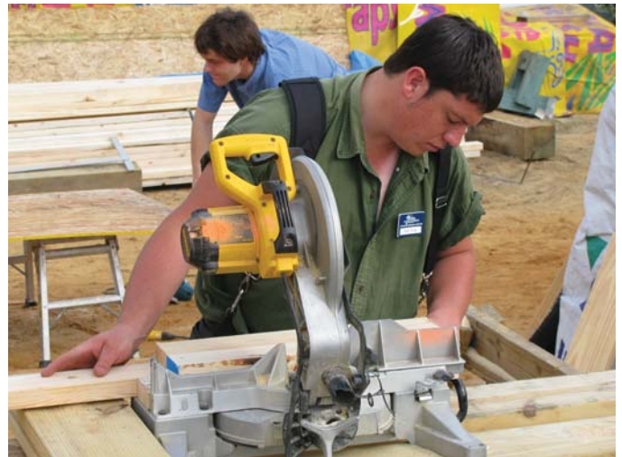
(FIG.A) DIMENSIONAL LUMBER is the most typical material used in residential construction due to its ease of construction, familiarity, and relatively low cost.
