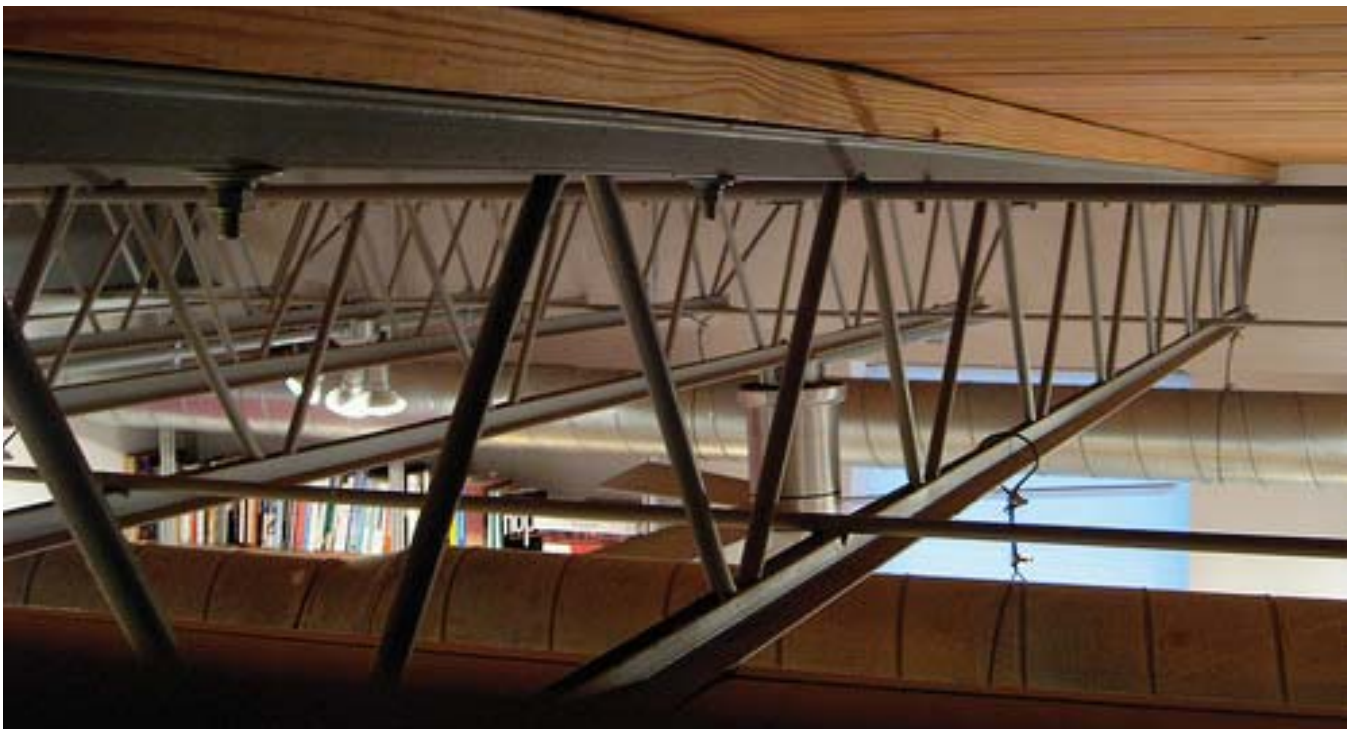
(Fig. 21) An engineered steel truss in a hybrid application.
