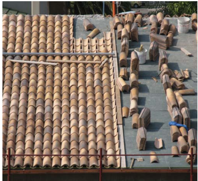
(Fig.17) Tile roofs require a thicker roof deck to support the added weight of the tiles. These tiles are being installed using mortar to hold them in place.
