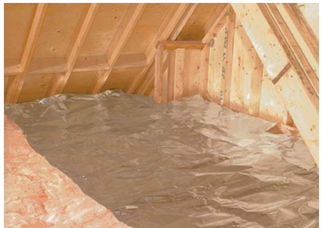
(Fig. 3) Rolled-out foil covers the attic floor insulation. Little fastening is needed to keep the product in place. Note the reflective side faces the interior.
