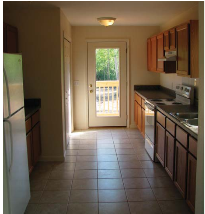
(Fig.19) Tile flooring is a durable, easy to clean choice for kitchens, bathrooms, laundry rooms, entryways, and other areas.
