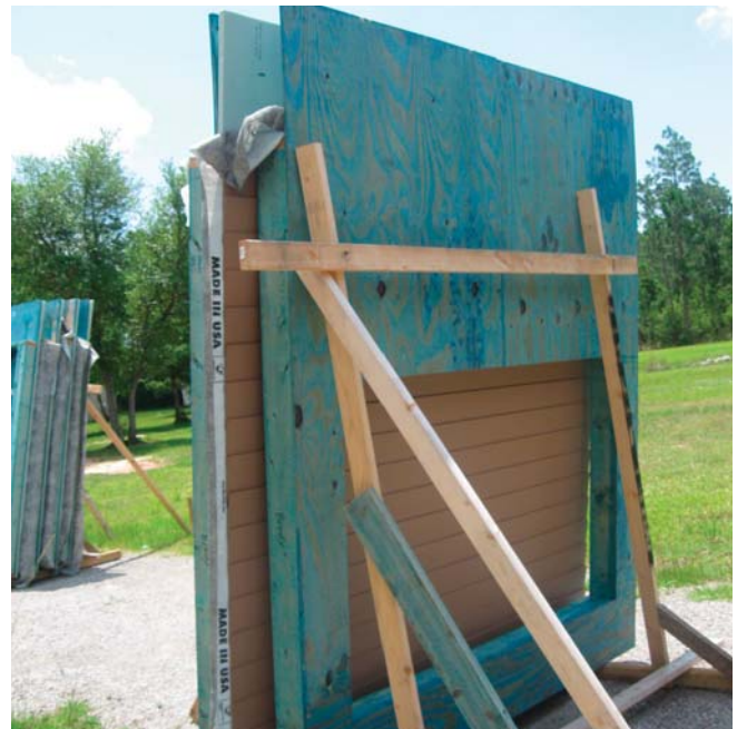
(Fig.16) Panel segments are delivered to the site already sided and with openings for windows.
