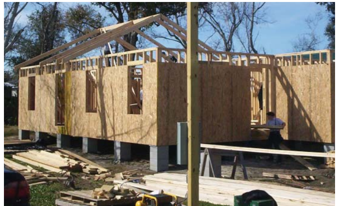
(FIG.B) SHEATHING creates a rigid building envelope, and helps resist shear forces. OSB sheathing is typically used on the Gulf Coast.
