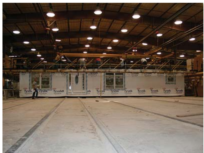
(Fig.5) Modular homes made in factories are made quickly with the help of specialized rigging and equipment.
