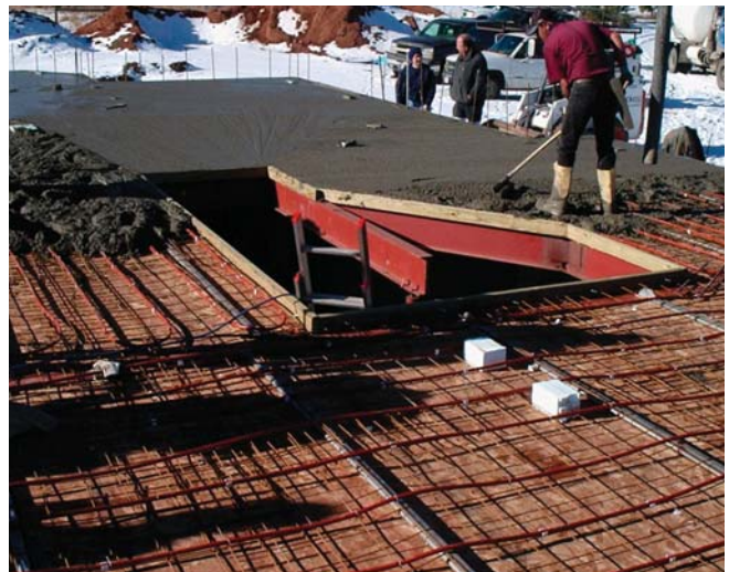
(Fig.8) A professional concrete installer spreads concrete over the formwork. Here, rebar is used instead of steel mesh for reinforcement.
