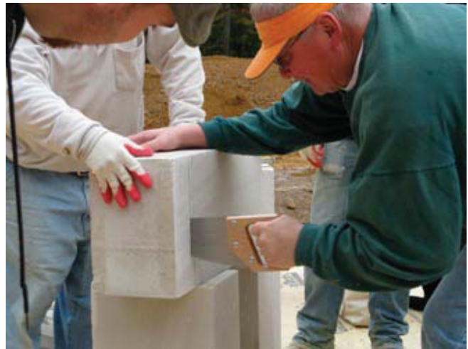
(Fig. 17) AAC blocks are easily cut on-site without the need for special saws or blades.
