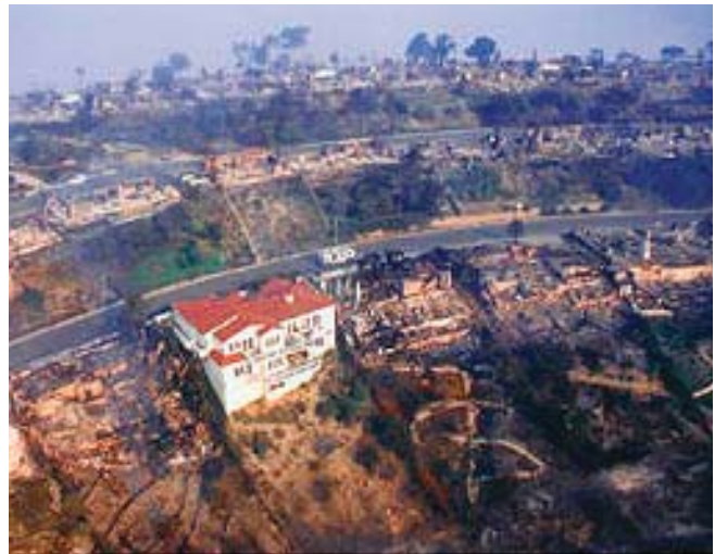
(Fig. 16) This AAC constructed house survived a wildfire. AAC blocks are highly fire-resistant.
