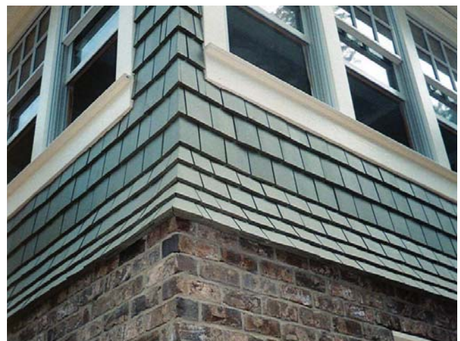
(Fig.10) Brick is used to accent the cypress siding above. Cypress is another popular wood species used in siding because it is water resistant.
