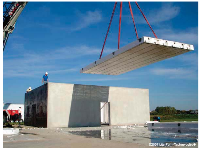
(Fig.25) A crane is used to lift panels into place.
