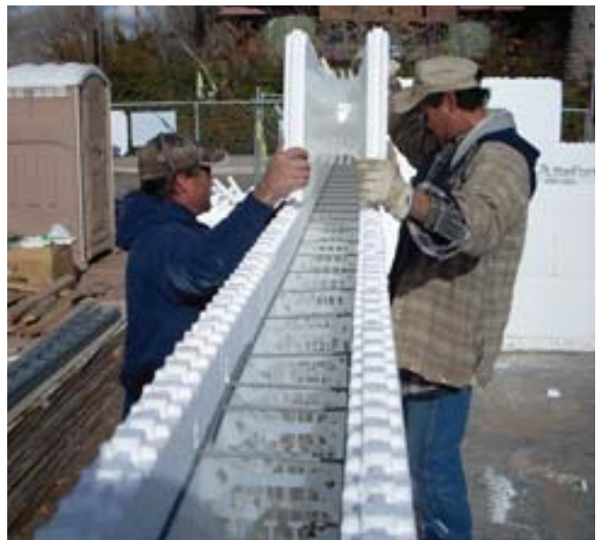
(Fig. 4) A small crew of just a few laborers is needed to stack the formwork.
