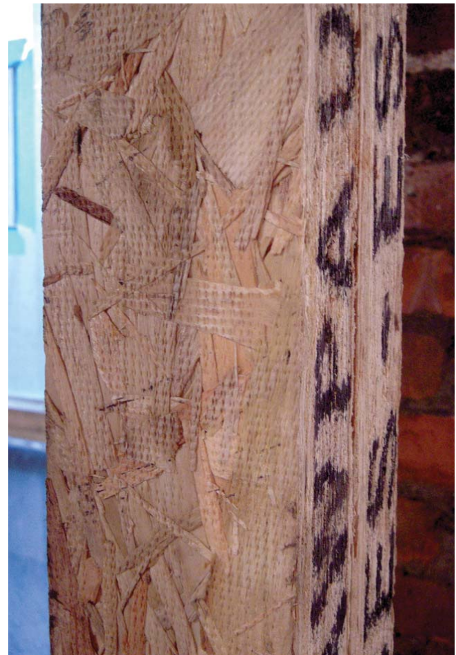
(Fig. 12) A close-up of an engineered wood stud.
