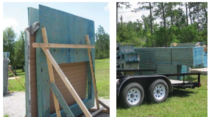
(FIG.C) KIT HOMES are delivered on-site with various parts to assemble. Included in the kit should be all the pieces needed to assemble the home.
