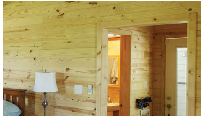
(FIG.D) INTERIOR FINISHES influence the comfort and versatility of walls. Tongue and groove pine boards (above) are durable and provide additional shear strength for the building. (photo © Alan Karchmer)
