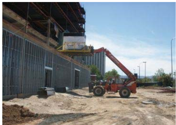
(Figs. 6-8) Component pods are delivered by truck and lifted into the structure.
