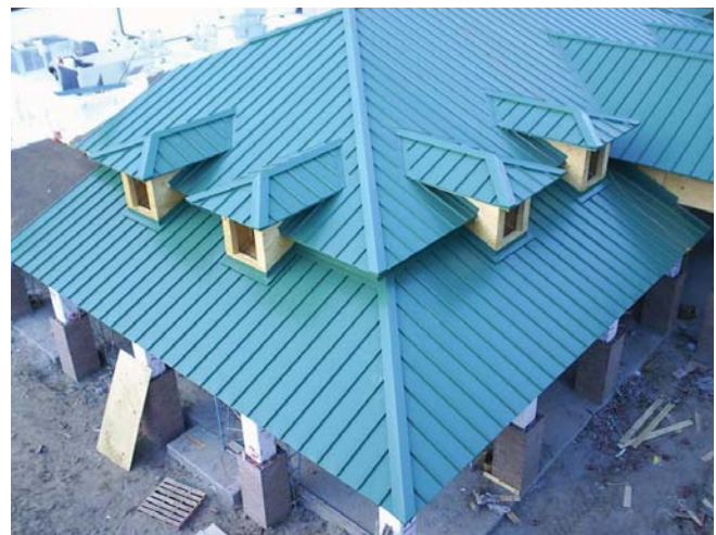
(Fig.15) Standing seam metal roofs are less common and more expensive, but have a longer life span.
