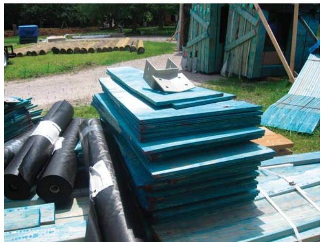
(Fig.14) The kit home construction observed as part of this research was a Deltec home. All the materials for the structure and the weather-proofing are included in the kit, but interior finishes are not.
