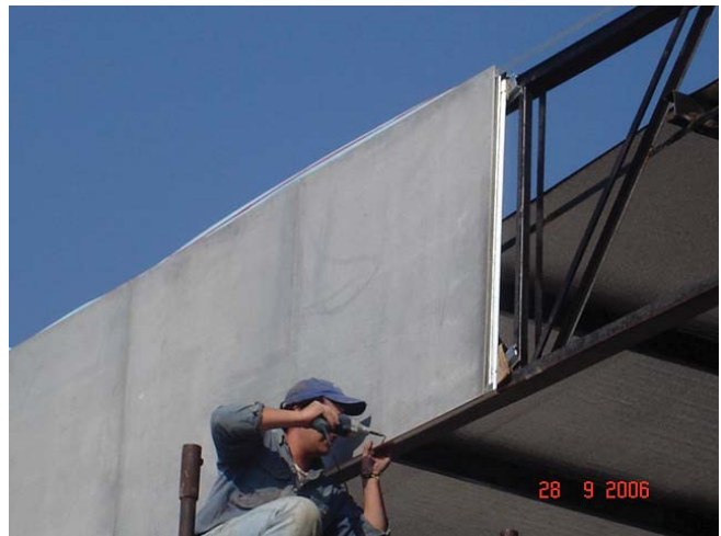
(Fig. 28) Magnesium oxide panels are used as the exterior sheathing in this building.
