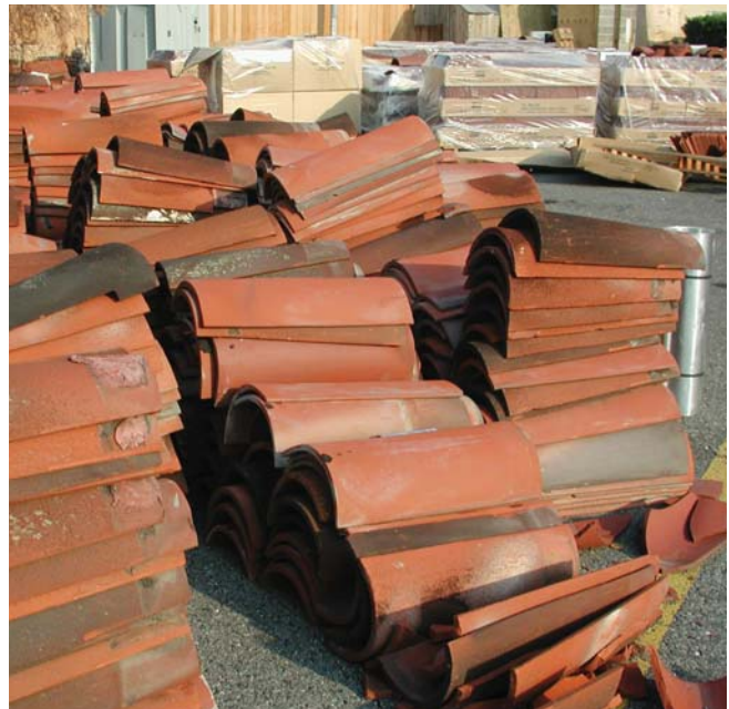
(Fig.16) Tile will be delivered to the site on pallets. The weight of tile makes them difficult to move around on site.
