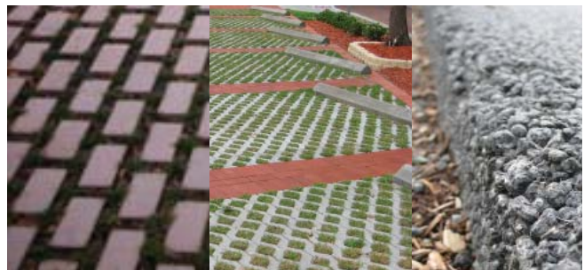
(Fig. 7) Porous paving systems are available in many different forms and materials, which allows for flexibility in choosing the right paving system for each project.
