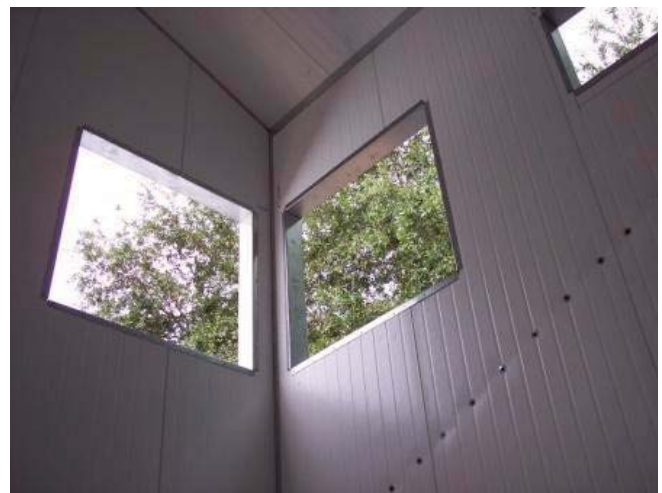
(Fig.16) Metal SIP corner showing window openings cased out using galvanized steel channels.
