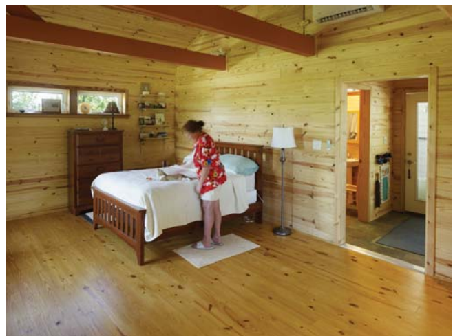
(Fig. 32) Solid wood, such as this 2x6 tongue-and-groove southern yellow pine, is a durable and natural finish for a room.
