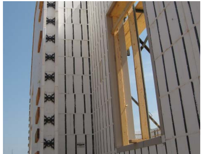
(FIG.A) INSULATED CONCRETE FORMS (ICF) is often manufactured with plastic vertical strips for adhering exterior finish material.
