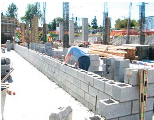
(Fig. 13) CMU walls are often used for exterior walls, in combination with interior wood stud walls.
