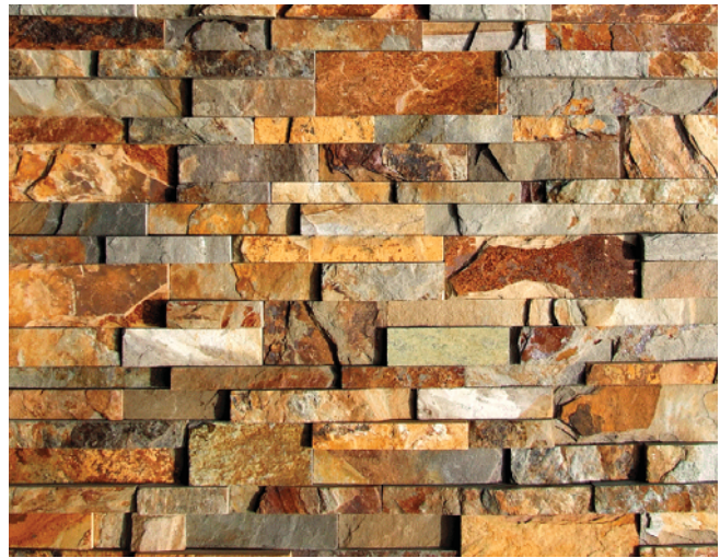
(Fig. 36) Cast stone is made to replicate the appearance of natural cut stone.
