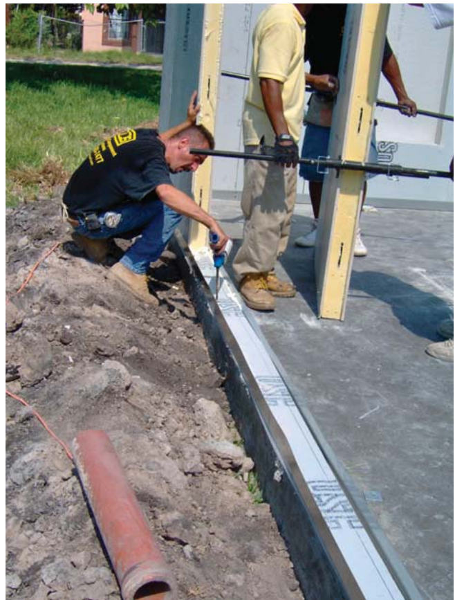
(Fig.14) A worker installs fiber cement panels in a house in Orlando, FL.
