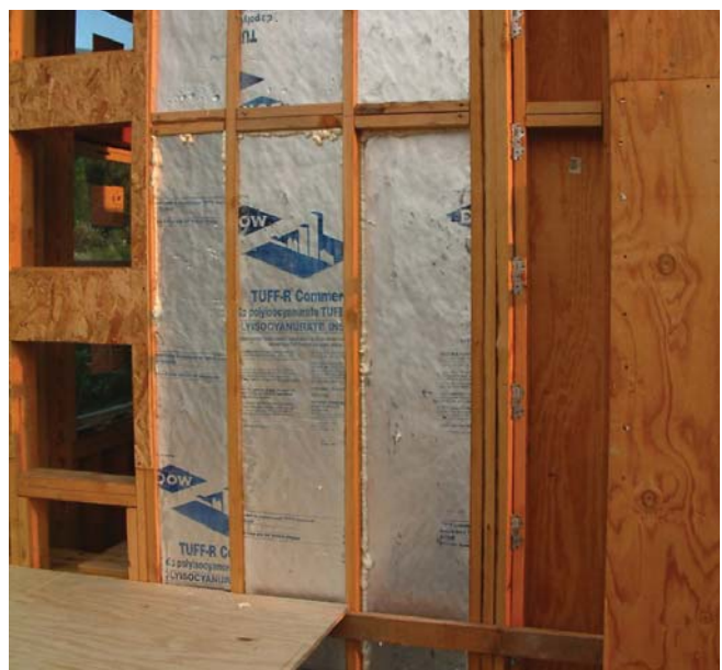
(Fig. 7) Radiant barriers are commonly used in the attic, but can be installed in other locations. This image shows radiant barrier backed plywood being used inside a wall cavity.
