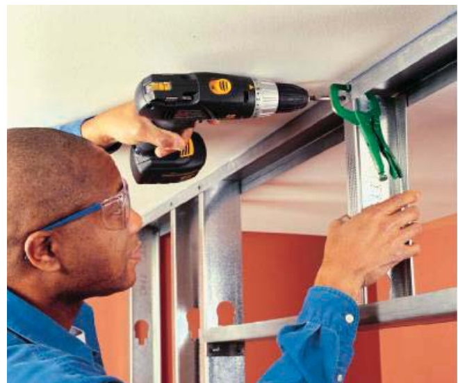
(Fig. 14) After setting the guide tracks the studs are attached to create the walls.
