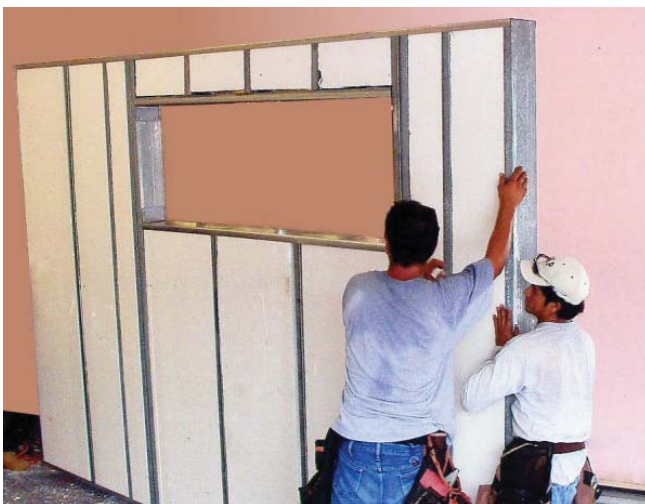
(Fig.20) These panels, manufactured by Dynabilt, combine galvanized steel framing with a polymeric insulated core.
