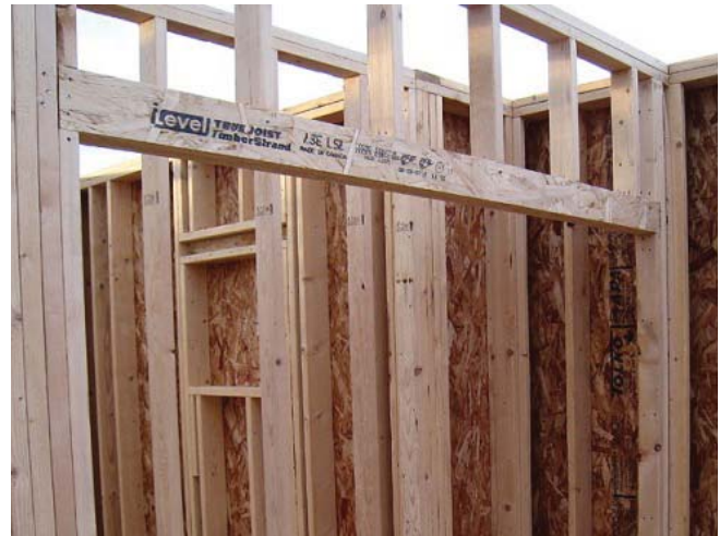
(Fig. 10) An LSL used as a header along with typical wood frame construction.
