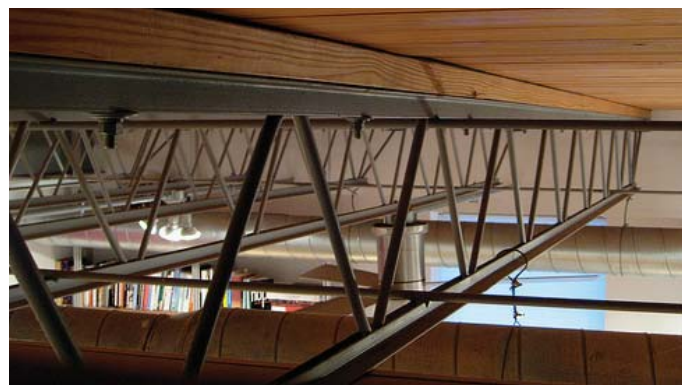
(FIG.C) TRUSSES offer a speedy alternative to traditional lumber joists in both floor and roof systems bridging larger spans and flexibility in the running of MEPs.
