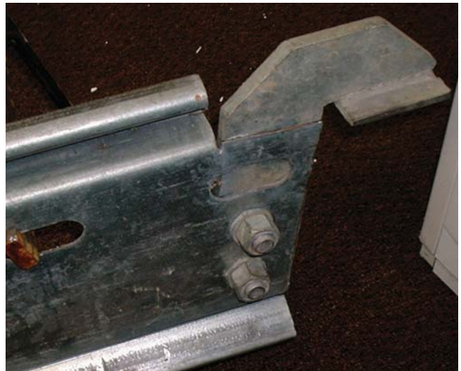
(Fig.6) Steel joists are anchored to foundation walls with an extended shoe (as shown above) that is then set into concrete.
