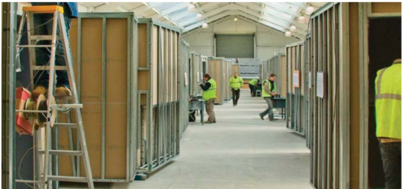
(Fig.9) Pods can be easily wired and plumbed due to greater access and a factory setting which encourages quality and efficiency.
