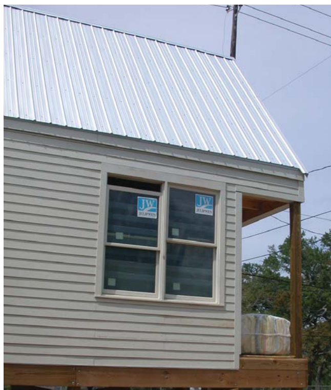
(Fig.12) Sheet metal roofs can handle slopes from 1:12 to nearly vertical, and are a good choice in sunny climates.
