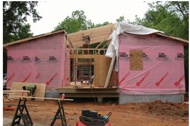
(Fig.19) Auburn University's DESIGNHabitat students work on a project that is an example of how on-site construction can combine pieces of factory-assembled modular homes to create a hybrid home.
