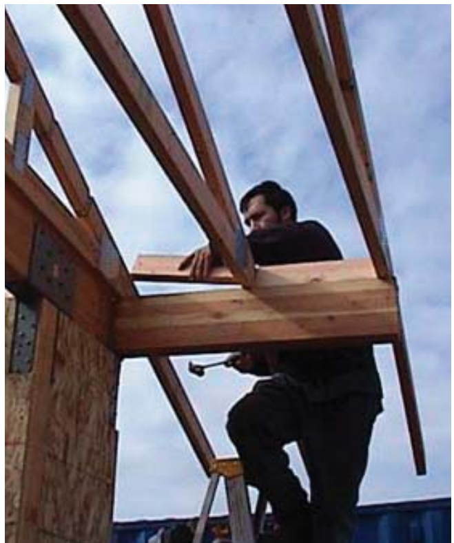
(Fig. 23) Blocking is nailed in place to tie the trusses together.
