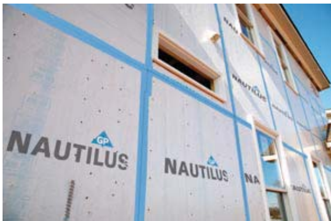
(Fig. 16) Nautilus wall sheathing by Georgia Pacific is an alternative to OSB and Plywood. It is produced with a moisture barrier pre-affixed and has begun to gain favor among builders.
