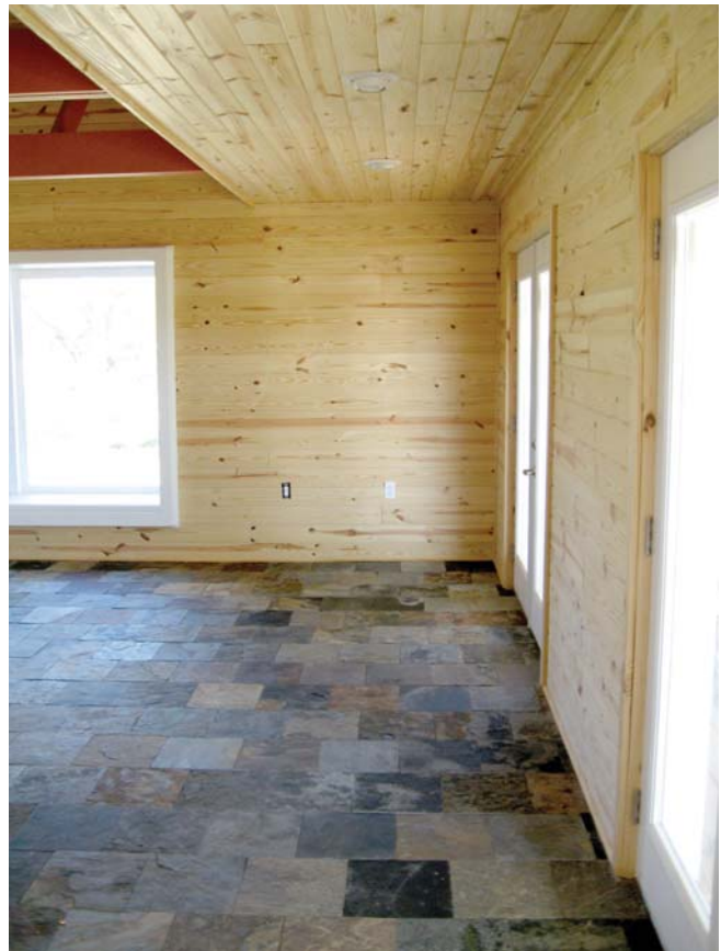
(Fig.23) Stone flooring, such as slate tile shown here, can be beautiful and durable. However, slate can be hard to clean and can stain if not properly sealed.
