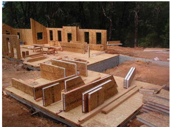
(Fig.2) Panels laid out on a building site prior to erecting the walls. A partially assembled house is visible in the background.
