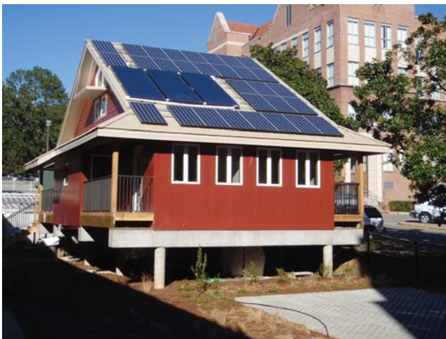
(Fig.8) Florida State University Energy & Sustainability Center’s “Off-Grid Zero Emissions Building”.
