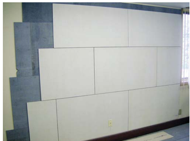
(Fig. 26) Magnesium oxide panels are considered to be more mold resistant than typical drywall.
