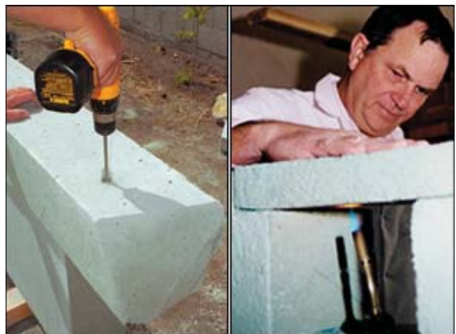
(Fig. 18) Vertical holes are drilled through the blocks for reinforcing bars. After the bars are set, the holes are filled with structural mortar.
