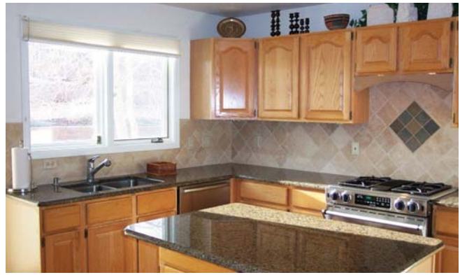
(Fig. 33) Tile used for a kitchen backsplash creates a durable and attractive surface and protects the wall from grease and moisture.
