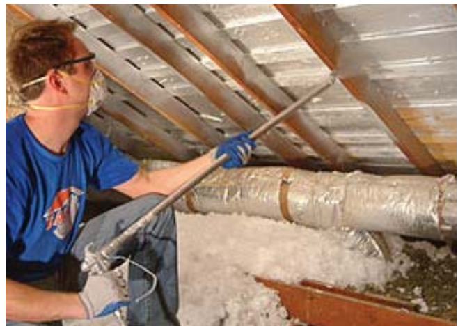
(Fig. 4) A spray-coated radiant barrier can be applied to the underside of the roof decking.
