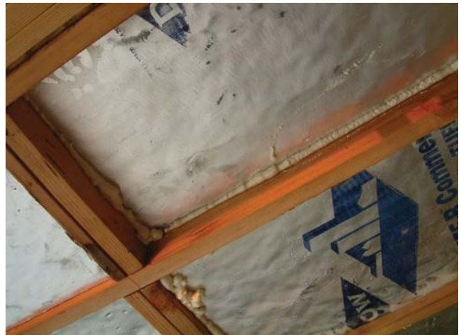
(Fig. 2) Foil backed sheathing can add radiant protection with no additional construction time. Note the shiny side faces the interior.
