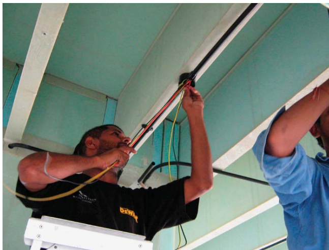
(Fig.15) A worker installs wiring in a house built using InnoVida fiber-reinforced plastic panels in Dubai, UAE.
