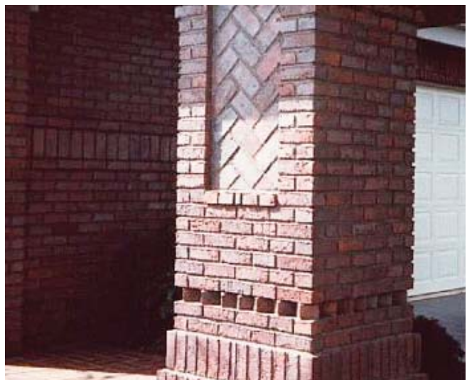
(Fig.3) With an experienced mason performing the installation, brick can be laid in a variety of patterns.
