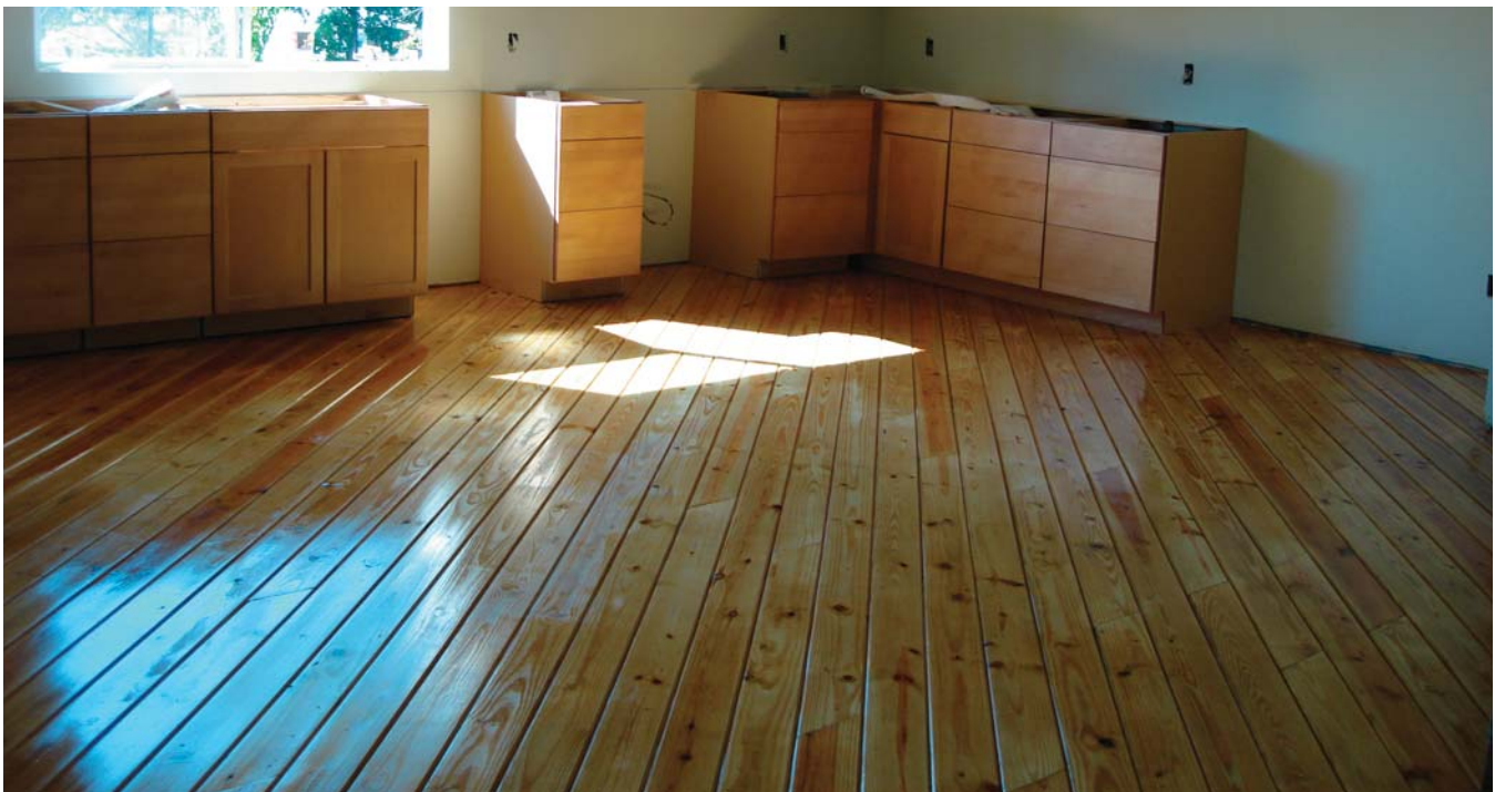
(Fig.1) 2x6 tongue and groove decking is simply stock lumber routed with tongues and grooves along its sides. Its additional depth makes it a strong and simple floor material.
