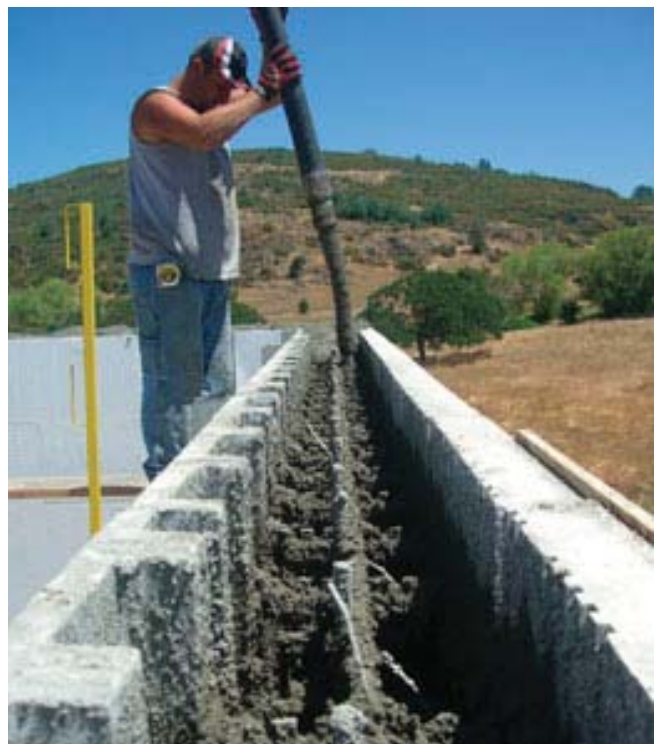
(Fig. 7) ICF walls are poured with concrete in 4' lifts, horizontally, with a concrete pump.
