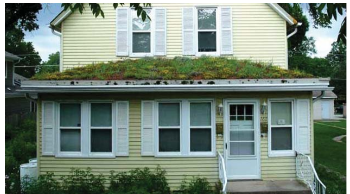
(FIG.C) Green Roofs are an unusual option in residential construction. The larger the area, the greater the insulative impact.
