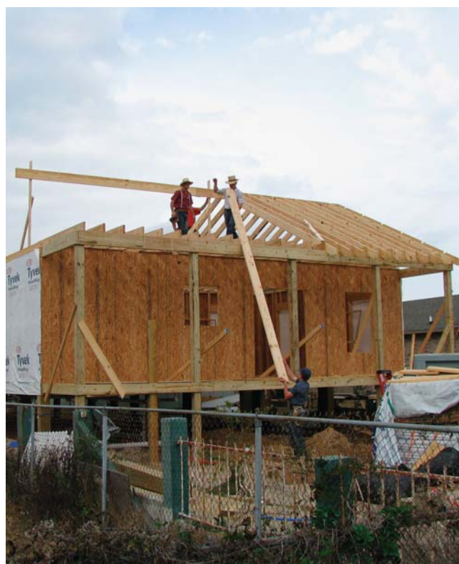
(Fig. 15) Properly nailing and wrapping the sheathing with a moisture barrier is essential to prevent rot and mold in hot and humid climates.
