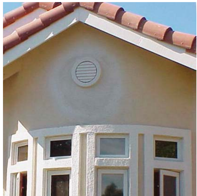
(Fig.5) Stucco can be applied in a variety of textures. Above, a smooth finish is used for the exterior wall, while a rough finish is applied to the window trim.
