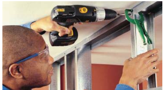
(FIG.B) STEEL STUD FRAMING is a viable alternative to dimensional lumber framing and in large volumes can provide cost savings for the builder.
