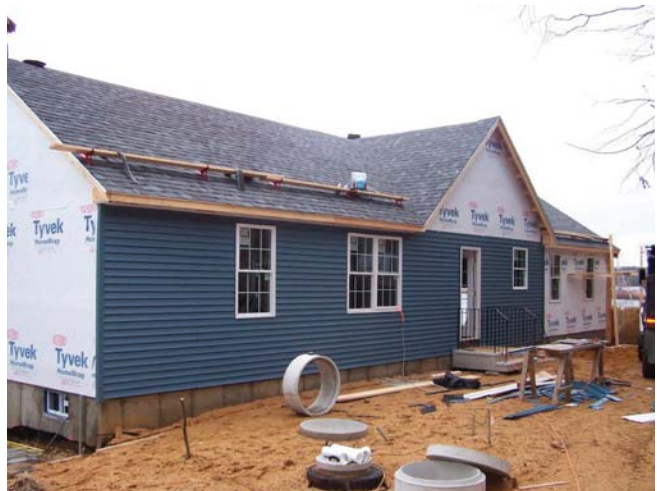
(Fig.2) Vinyl siding is designed to mimic wood planks, and is easy to install.
