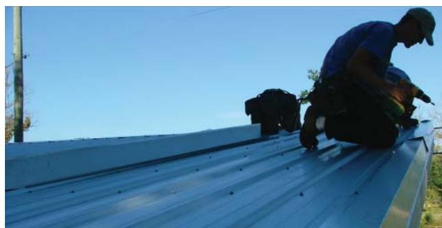
(Fig.11) After the sheet metal is in place, contractors install the top rake cap.
