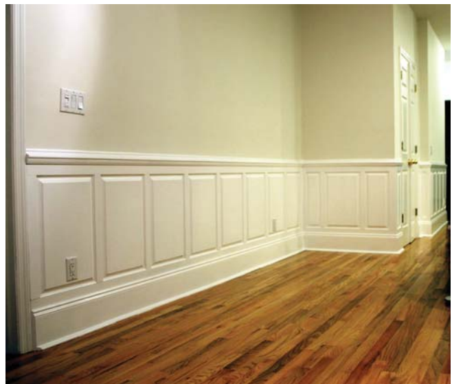
(Fig. 31) Wainscoting is a traditional application in which wood paneling (often painted) is used on the lowest 3' - 5' of the wall.
