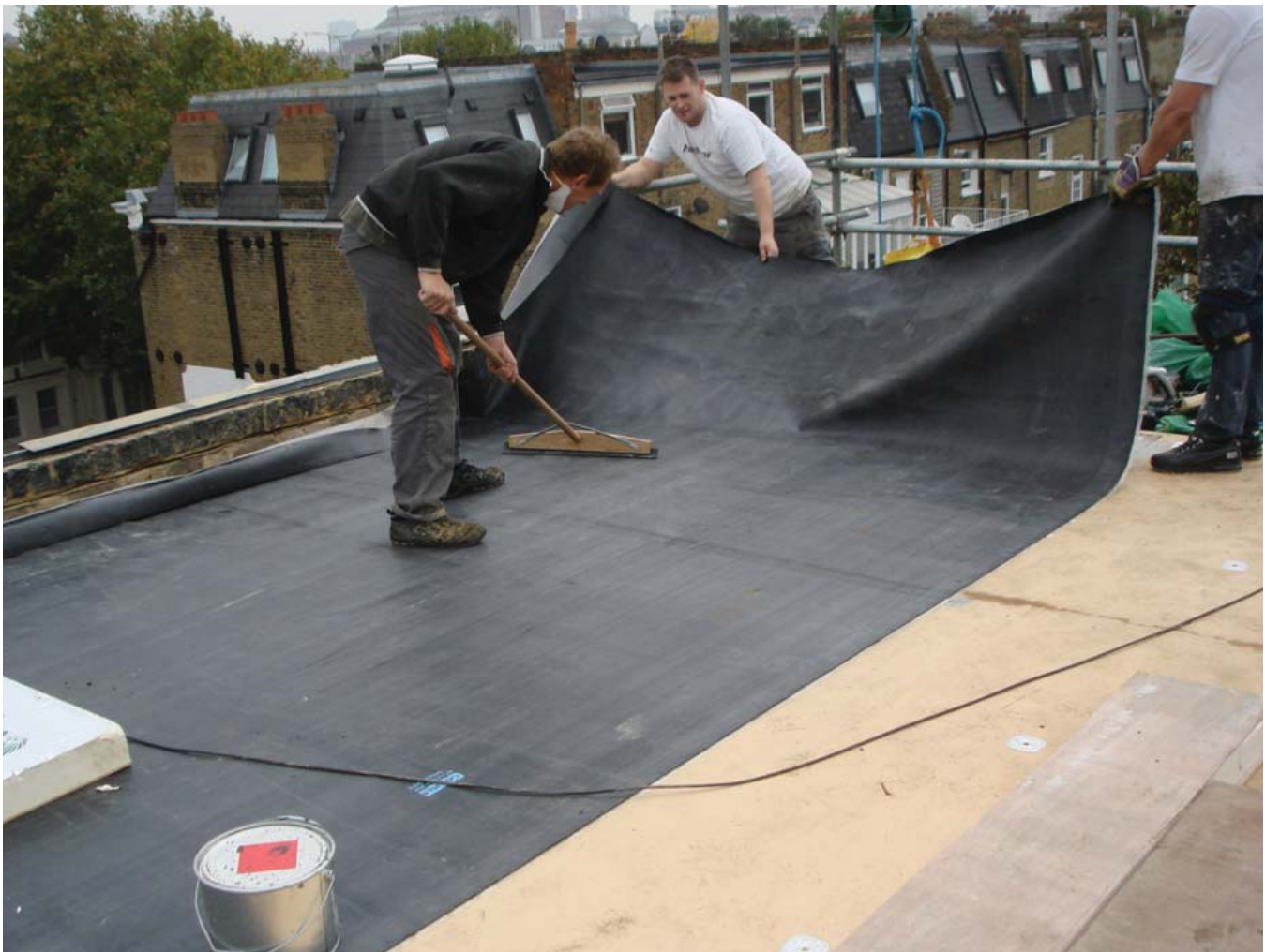
(Fig.21) Installing an EPDM roofing membrane is a relatively straightforward task, but requires care and the appropriate adhesives.
