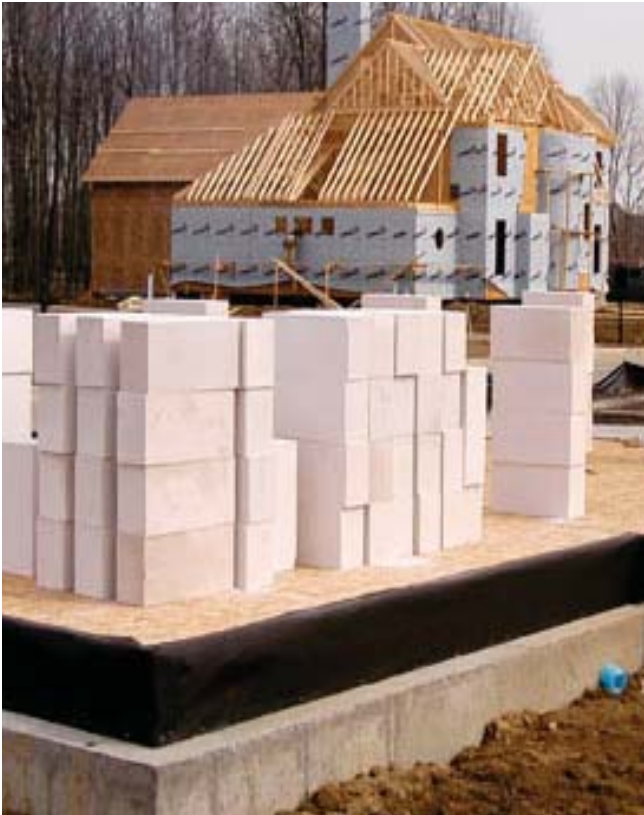
(Fig. 19) AAC blocks are easily brought to a site with lower shipping costs because they are lightweight.
