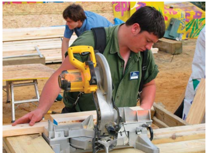
(Fig. 3) Basic carpentry knowledge is needed for wood frame construction.
