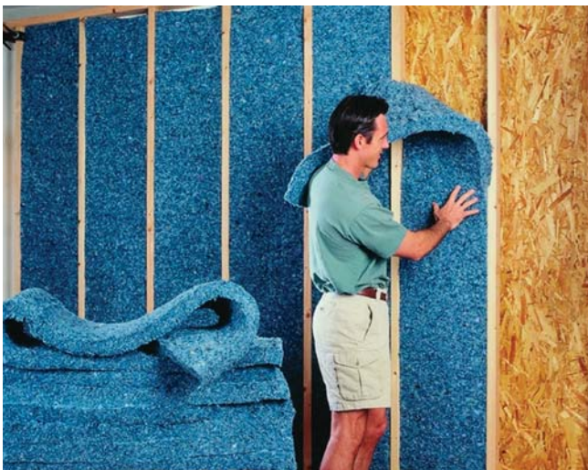
(Fig. 21) Cotton batt insulation can be installed without any special equipment or specialized labor.
